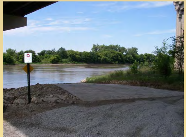
New 177 bridge river access and boat ramp
